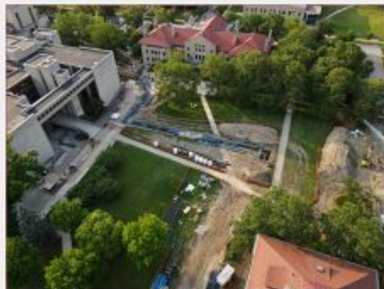
An aerial view of sustainable infrastructure work in Wilder Bowl. Photo credit: William Bradford
